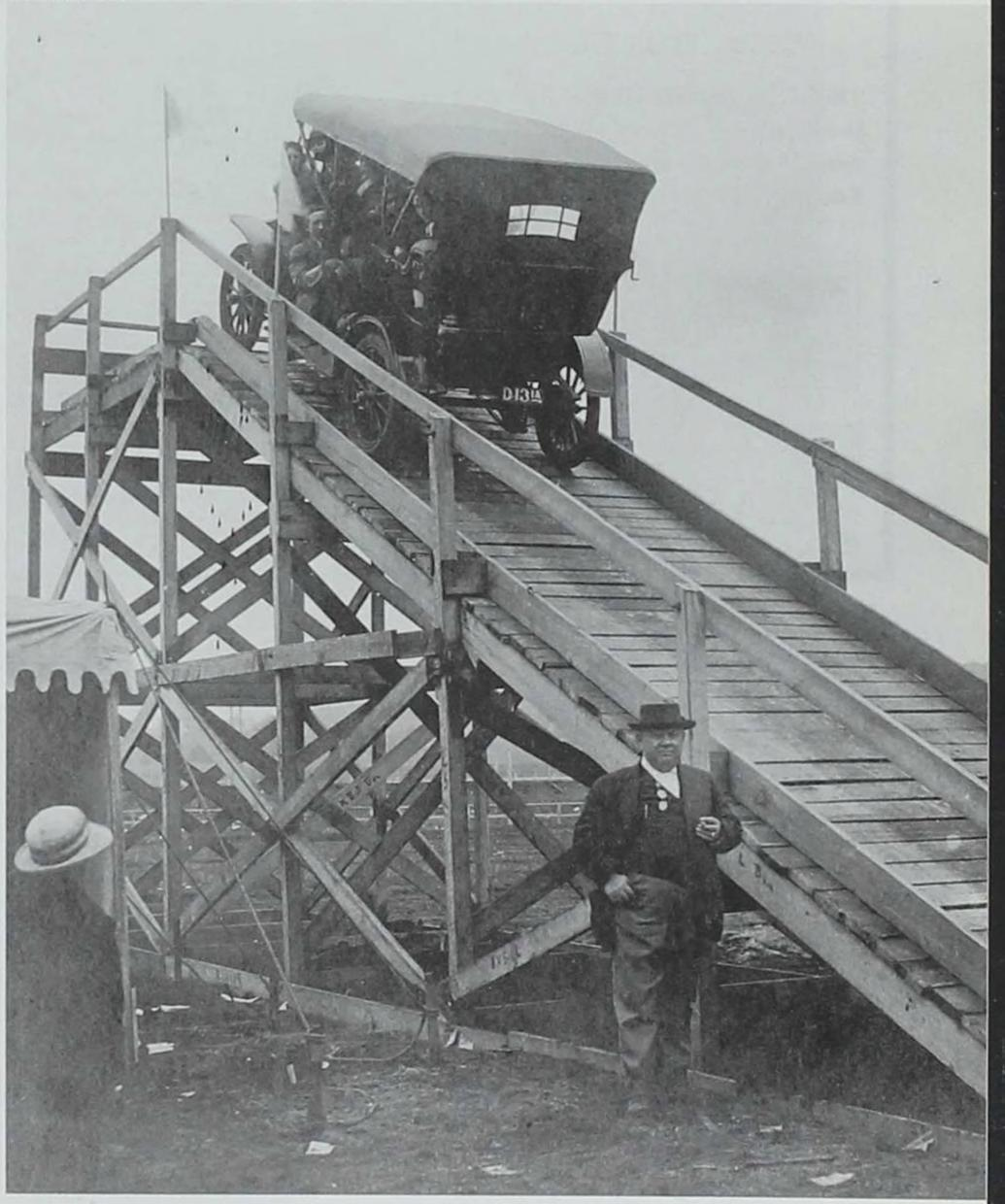
On a 50 percent incline set up near the 1909 Iowa State Fair, a Mason once again demonstrates why it was called the "hill climber." Eleven passengers are inside the vehicle, while part owner Edward Mason stands by the ramp.
