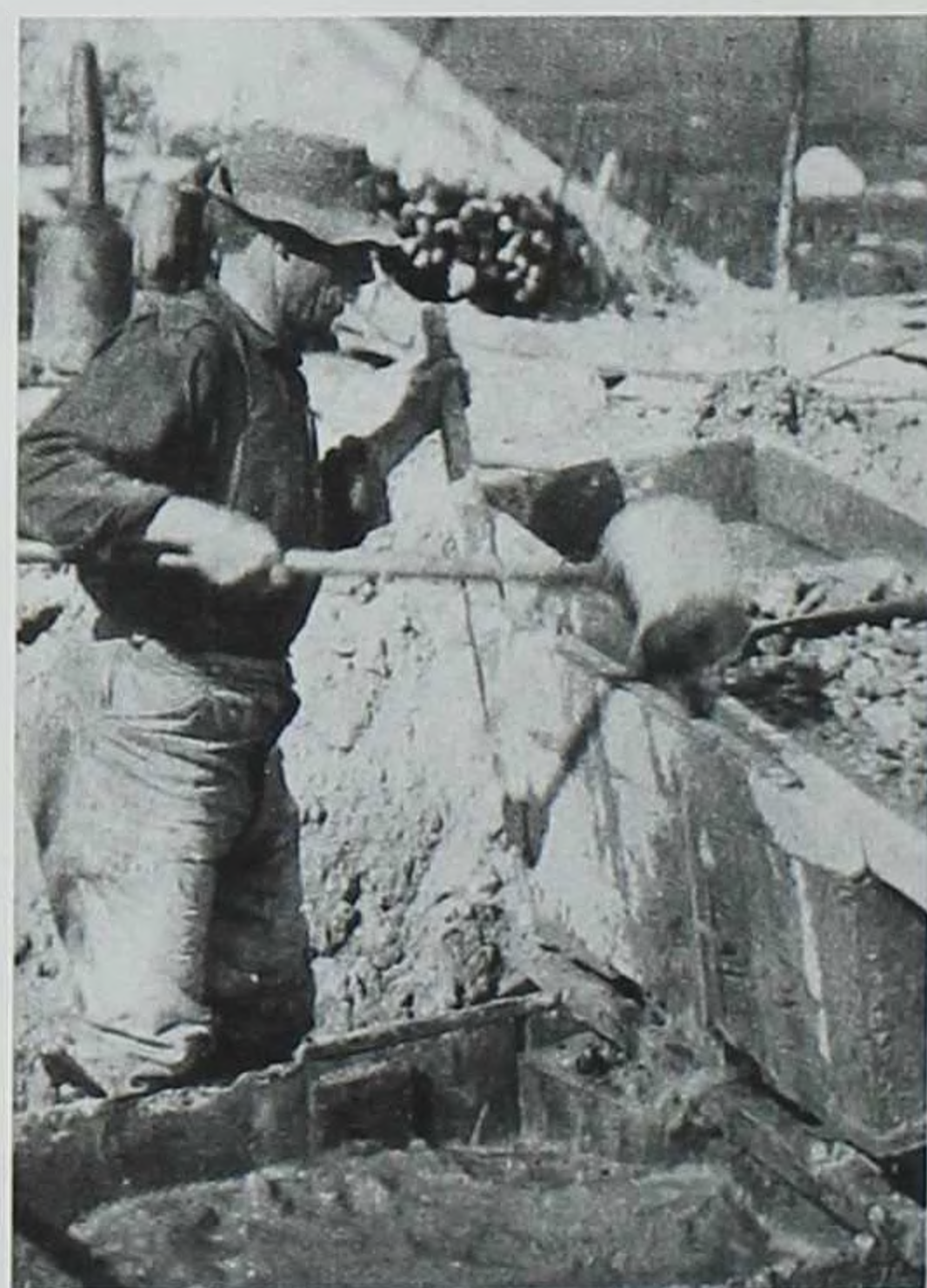
A miner pours water over gravel to loosen the gold, which next falls through a screen as the box is shaken.
