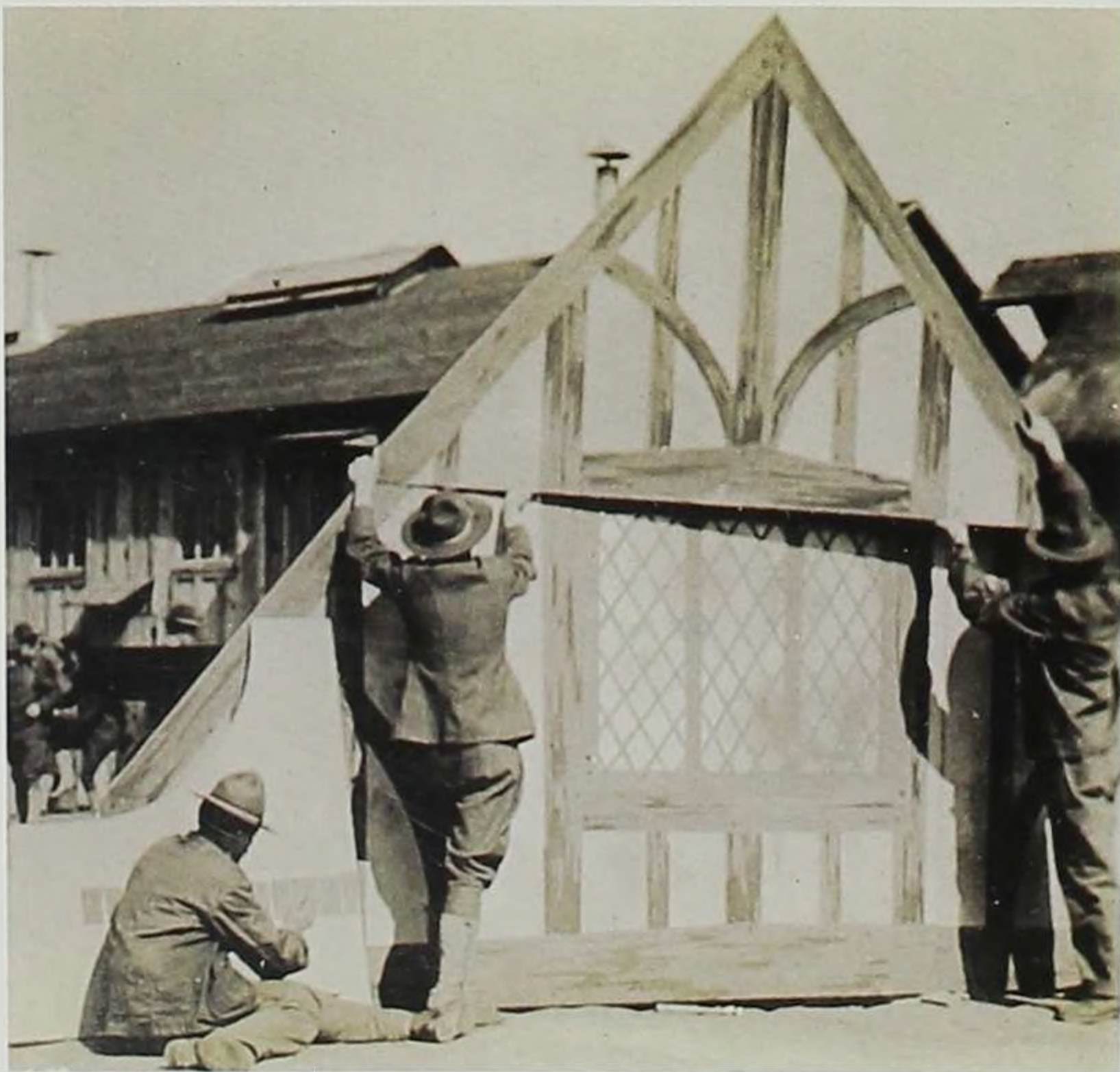
Men of the 40th Engineers of the American University erect a false house, its painted side resembling theatrical scenery.
