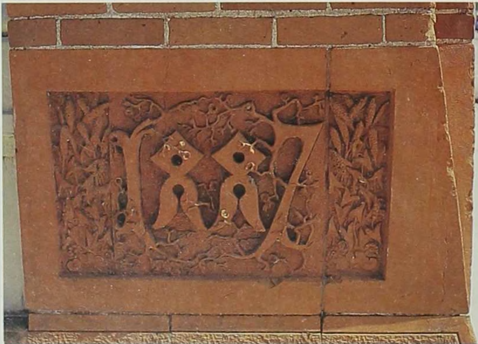
T erra cotta lent itself well to decorative flourishes, such as this cornerstone bearing the date construction began.
