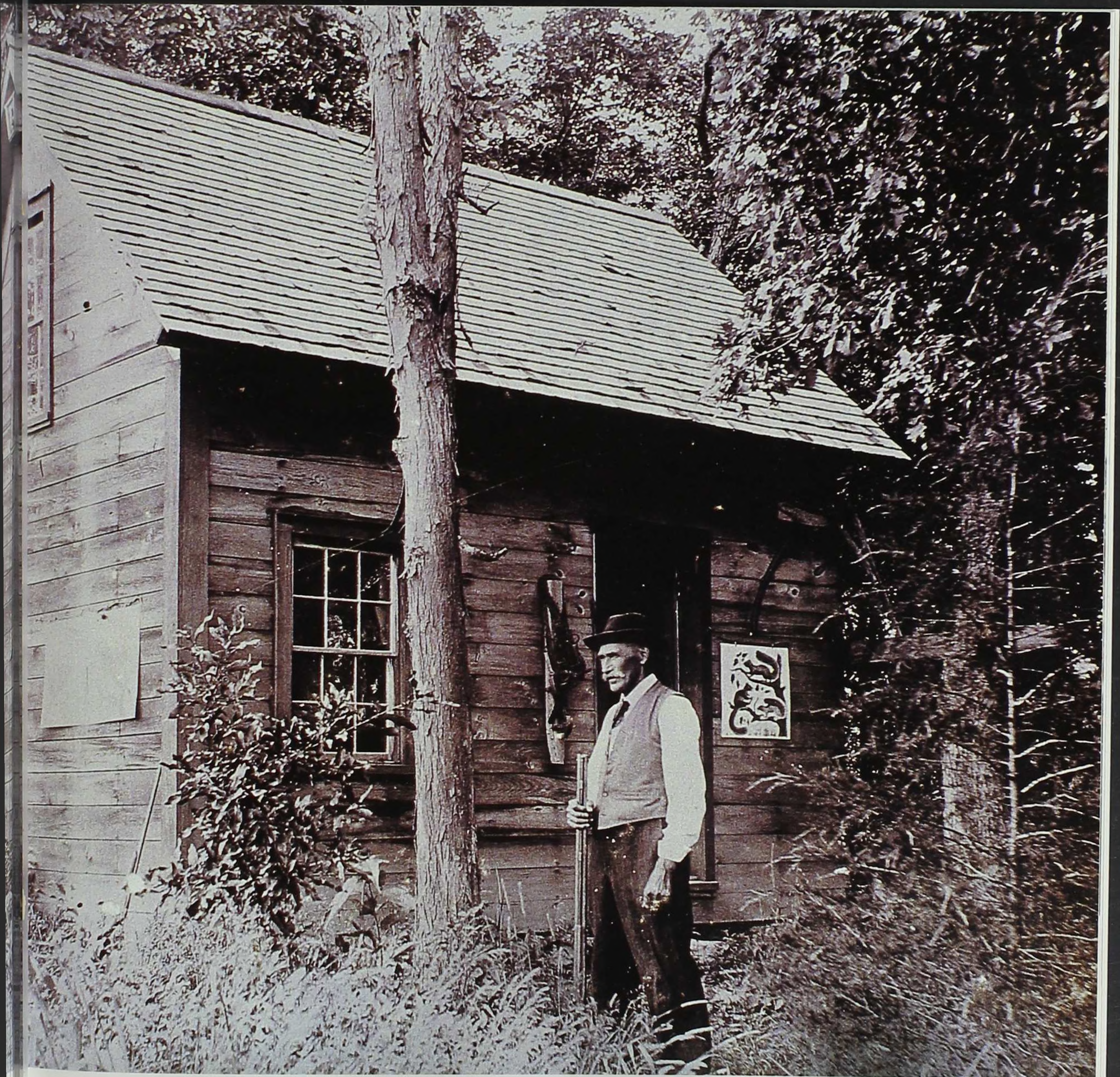
OFFICE EXTERIOR AND INTERIOR, SHSI (DES MOINES); ORIGINALS COURTESY OF LEWIS D. SAVAGE
