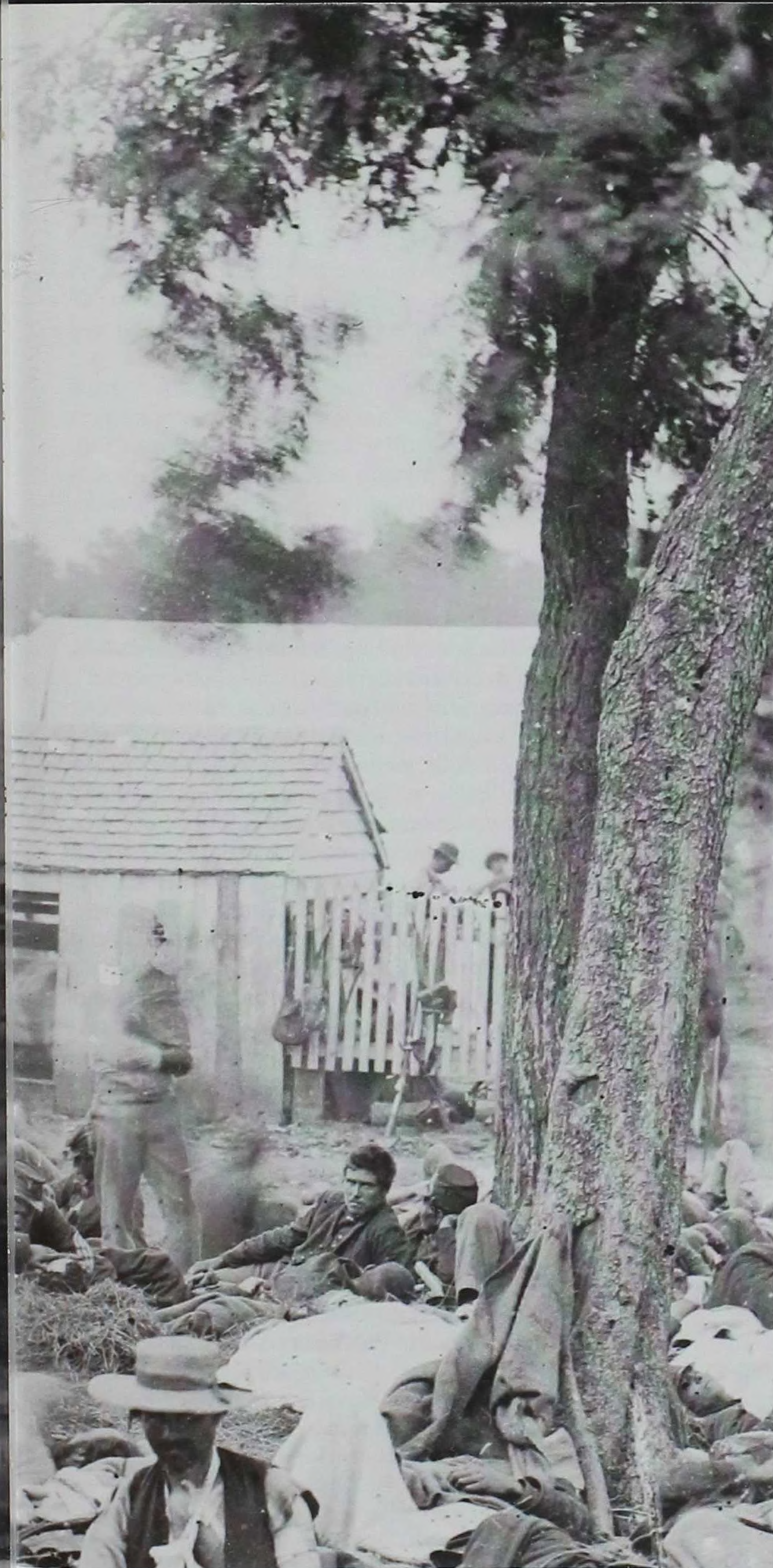
A field hospital in Virginia.
