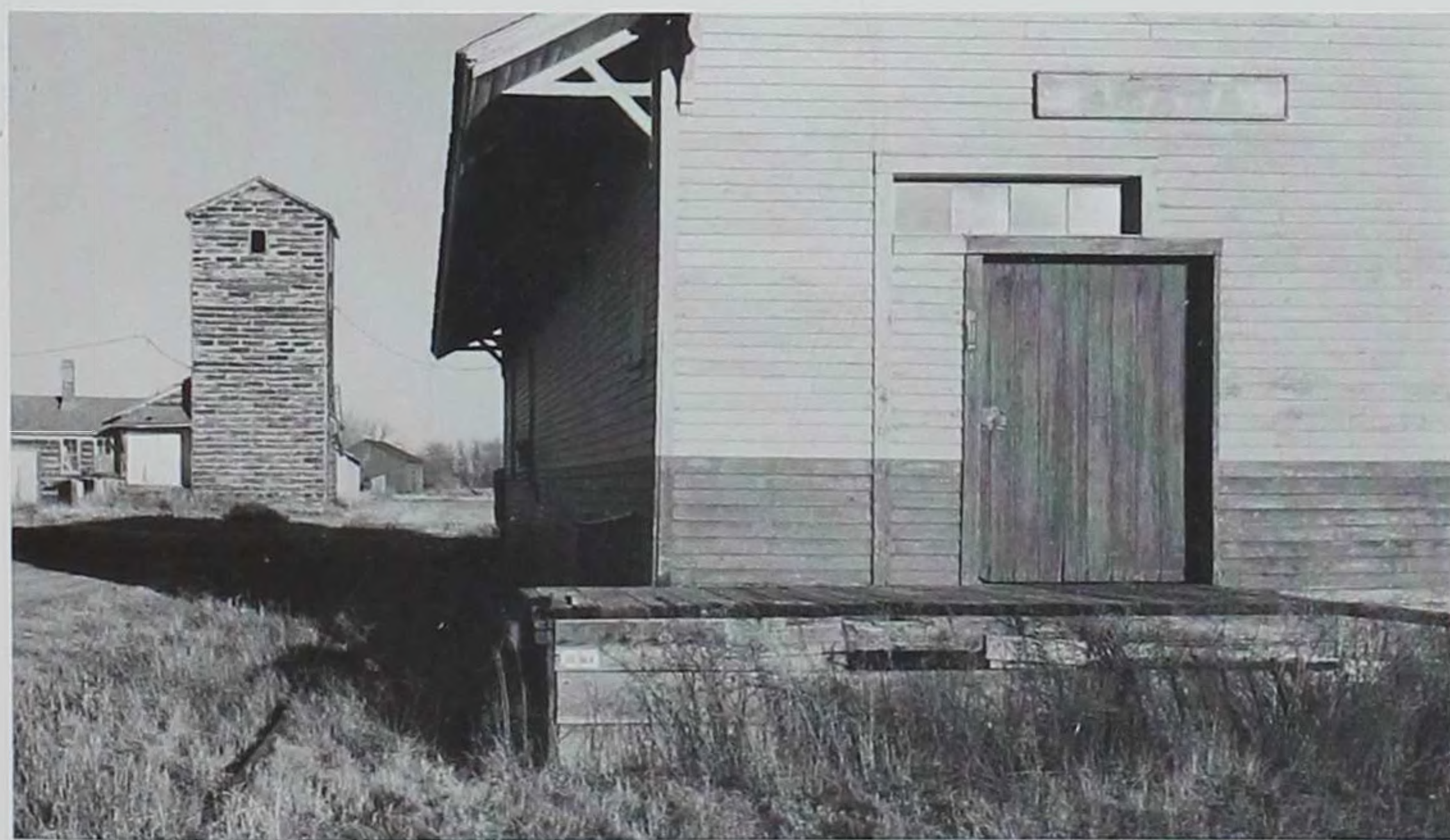
Above: Photographed in 1980, the Amana depot survived years of neglect, its brick platform stolen by souvenir hunters. Renovated by the Amana Preservation Foundation, it first served the Old Creamery Theatre and is now the trail head for the Amana Colonies Recreation Trail.
