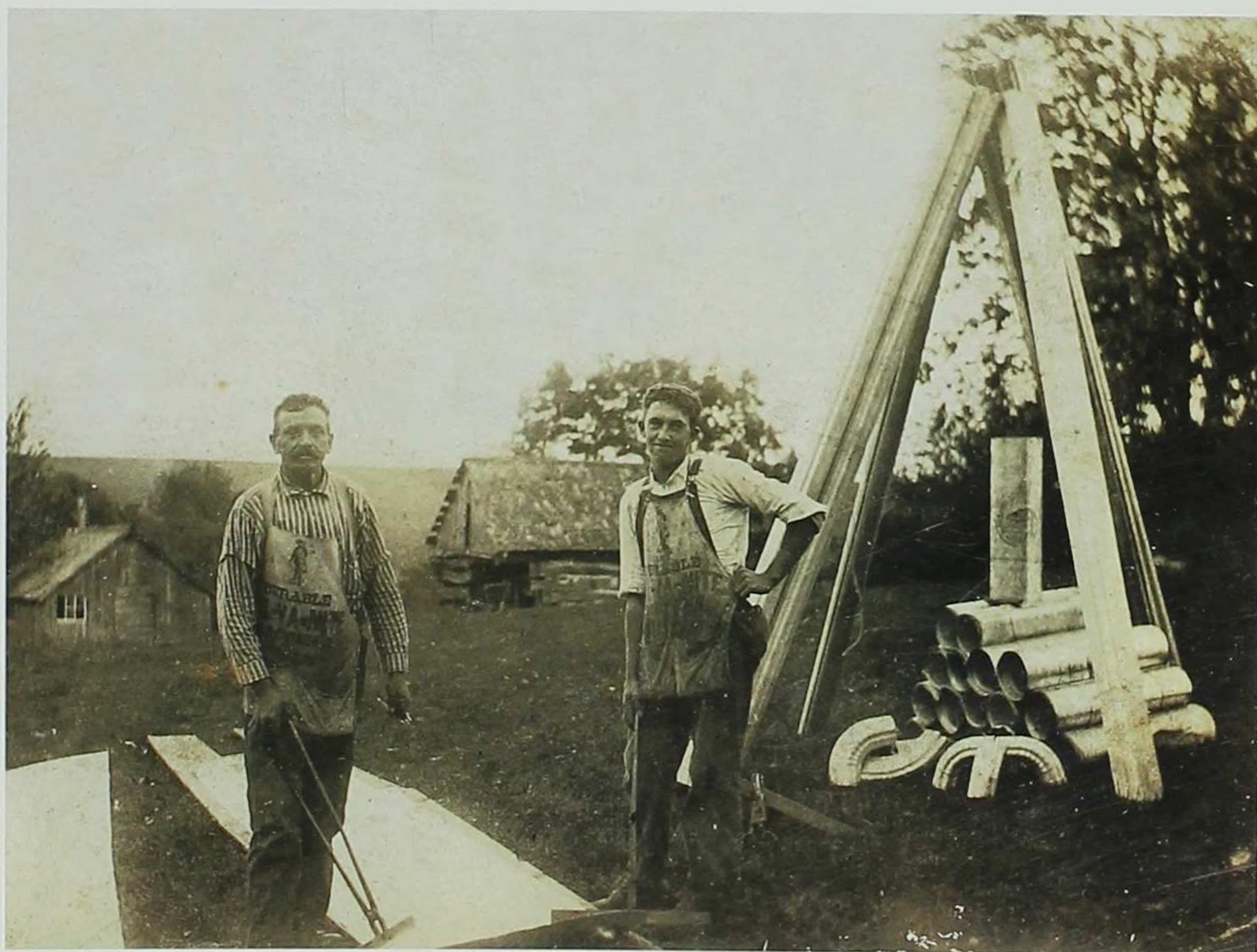
W ith hand on hip, Billy Bechtel stands beside a pyramid of gutters and downspouts. On the ground, sheets of tin await cutting and crimping.
