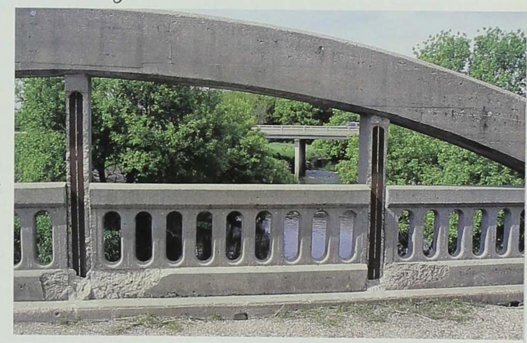
**B**uilt in 1914, the bridge on **Beaver Creek** (southern Union Township, Boone County) was replaced in 1996. Near right: Deteriorated concrete had left structural steel exposed on the arch ribs. Far right: Ice and logs during high water had damaged the arches' ends, where they were anchored to abutments.
