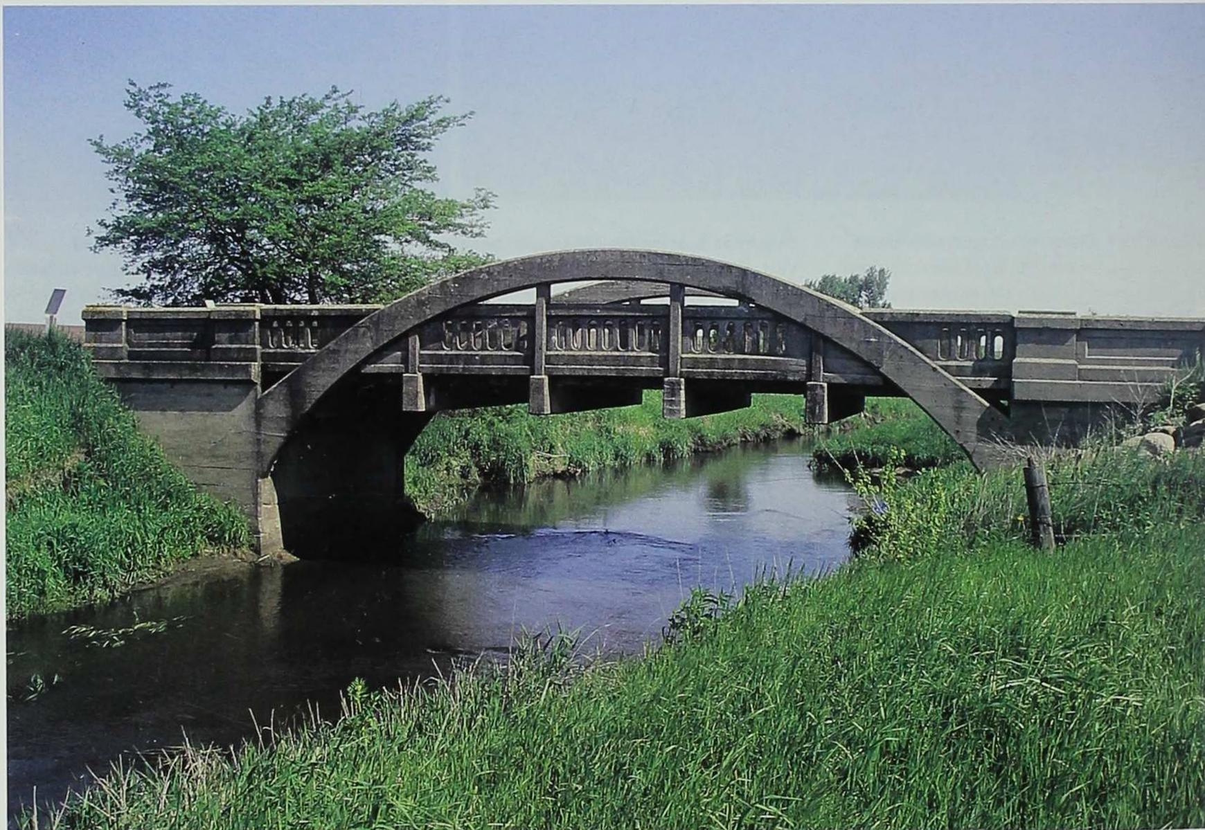
**A** Marsh Rainbow Arch bridge (built in 1916/17) crosses Big Creek (North) in Garden Township, Boone County. Note how the end of each arch tapers toward the abutment, and how the arch is anchored into the abutment below floor level.
