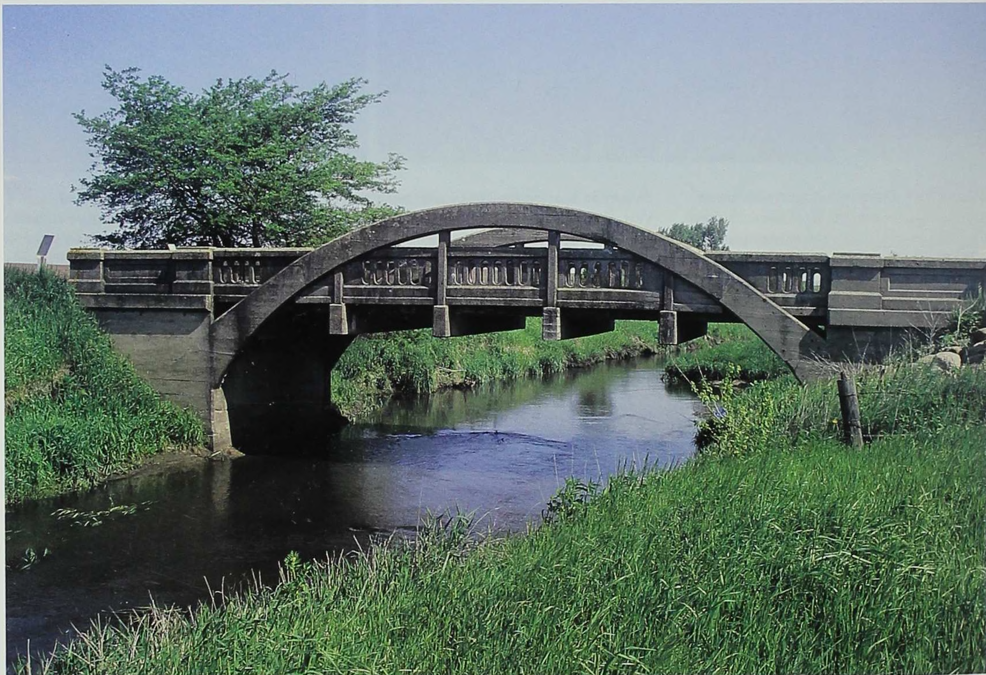
A Marsh Rainbow Arch bridge (built in 1916/17) crosses Big Creek (North) in Garden Township, Boone County. Note how the end of each arch tapers toward the abutment, and how the arch is anchored into the abutment below floor level.
