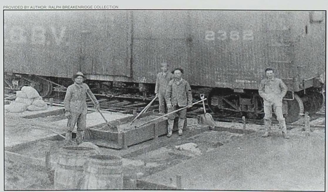
Several laborers take time to accommodate a photographer while they complete a cement floor for a storage building near the Fullerton Lumber Company yard in Macksburg. A boxcar immediately adjoins the construction site.
