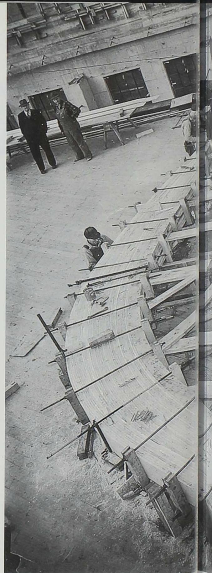
ing casein adhesive for strength. The glued lamination allowed roofs to span large open areas without the use of columns or other supports. By World War I, the use of timber arches had spread through Germany, Switzerland, and Scandinavia.
