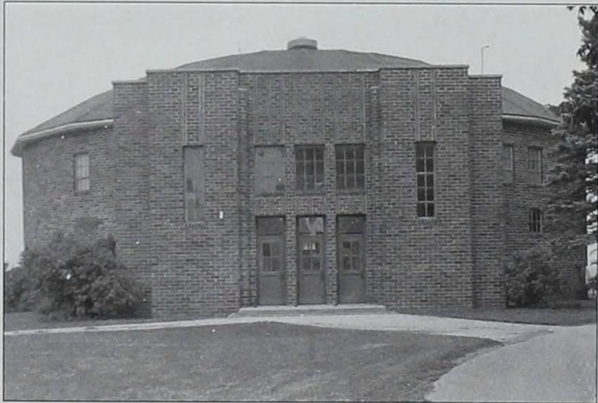
The New Providence school gymnasium is one of Iowa's few round gyms. The two-story building is constructed of hollow tile blocks with a brick exterior. The diameter is 85 feet. At its highest point, the low-pitched dome roof is 35 feet high and requires no supporting pillars because of the steel beam construction
