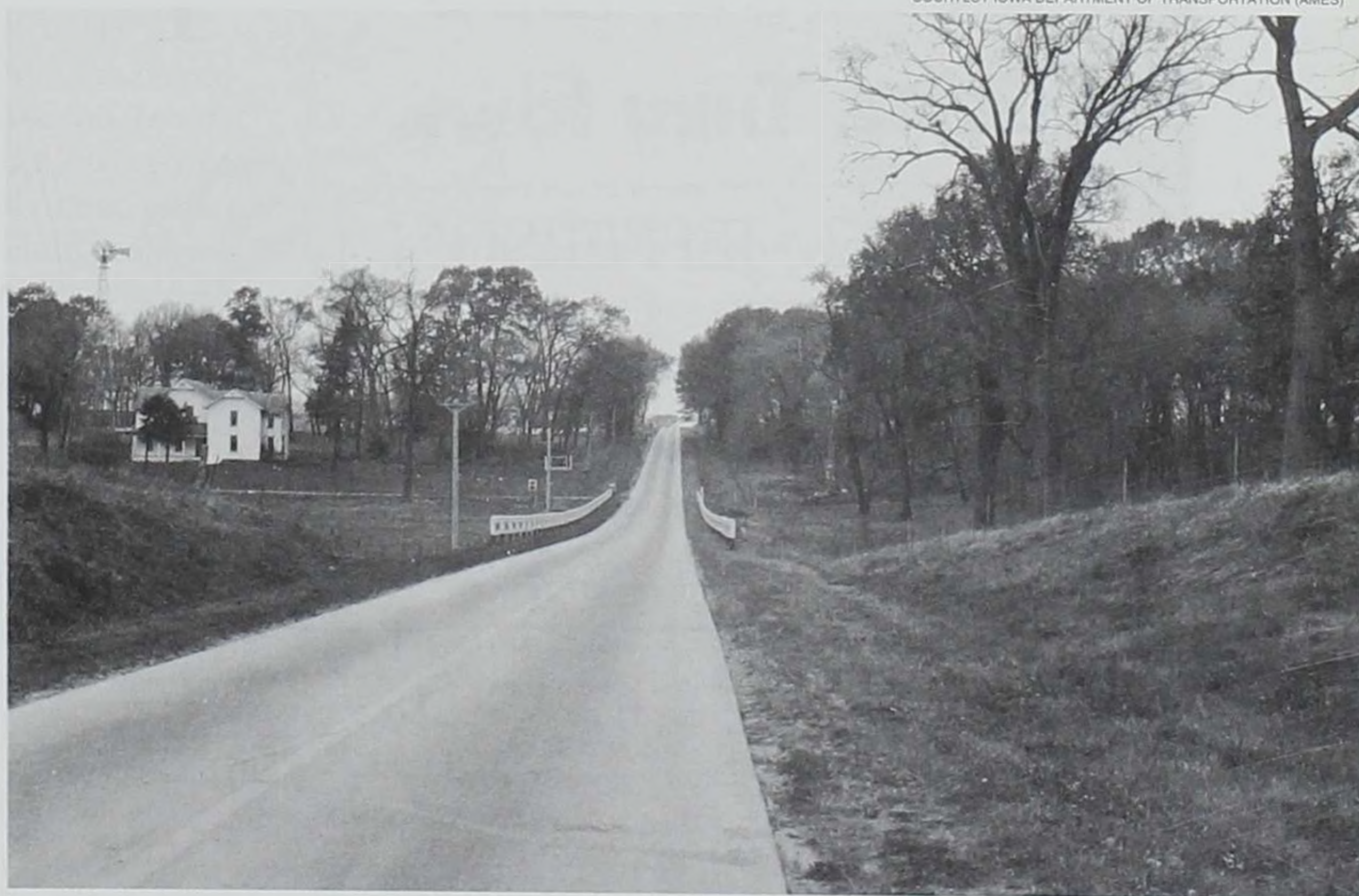
Above: Linn County's Seedling Mile heading northwest in 1928 offered a pleasant break from gravel. The 16-foot-wide ribbon of pavement was 200 feet short of a mile. In 1919, Greene County also paved a section of the Lincoln Highway, six and a half miles, with the help of federal funds.
