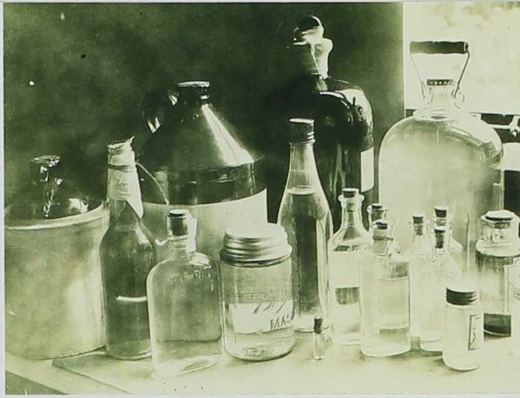
The Hygienic Laboratory repeatedly directed Iowans who wanted their well water tested to use the water collection kits provided by the lab (right), rather than salt-glazed jugs and bottles stoppered with corncobs, corks, or rolled paper (above)—all likely to contaminate the sample.
