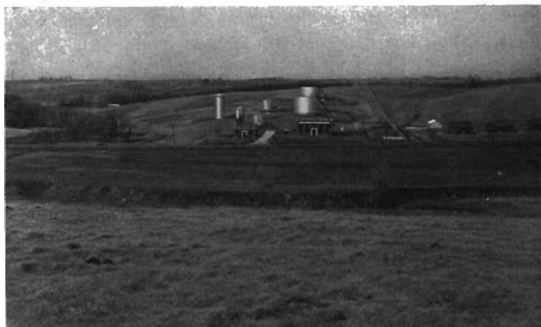
FIG. 24. — View of Great Lakes Pipeline Company Booster Station near Corning.
