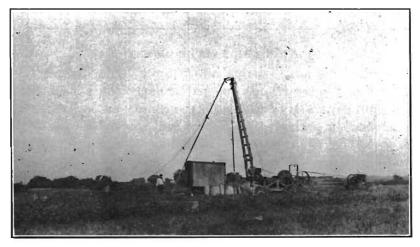
FIG. 22 .- Prospecting drill rig.
