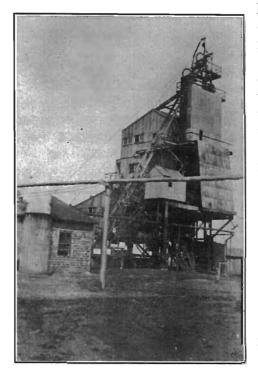
FIG. 27.-Tipple of mine No. 4.
