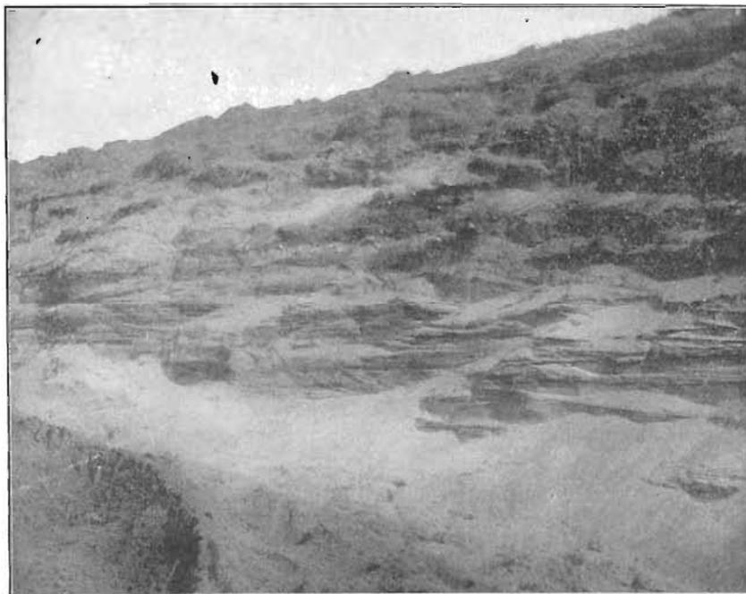
FIG. 16. The gravel pit of the Minneapolis & St. Louis railway, Estherville, Iowa. This illustration shows in a marked degree the characteristic cross-bedding of glacial gravels.
