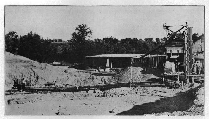
PLATE XLIX—Hammen pit showing belt conveyor, elevator and screen, Sac City Cement Pipe Company, Sac City, Sac county.
