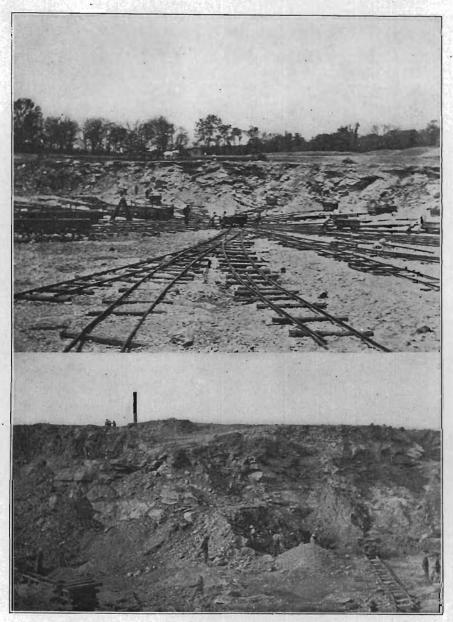
PLATE LII—Clark quarry, near Buffalo, Scott county; upper view showing trackage arrangements leading to incline, lower view showing irregular beds and large amount of shaly talus.
