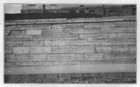
Fig. 62—Portion of retaining wall around Court House Square in Decorah, Winneshiek county, showing unreliable character of Galena limestone.
