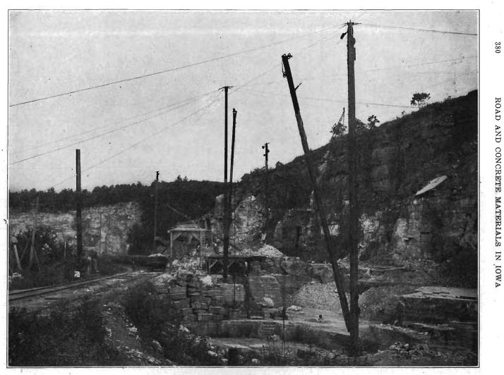
PLATE XXVI-John Ronen quarry, showing arrangement of tracks, derricks and crusher plant. Stone City, Jones county.
