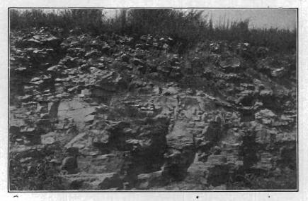
FIG. 64—Quarry in northern Lincoln township, Worth county, showing excellent material for road and concrete work.
