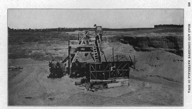
PLATE XLII-City gravel pit showing elevator and loading chute. Sibley, Osceola county.
