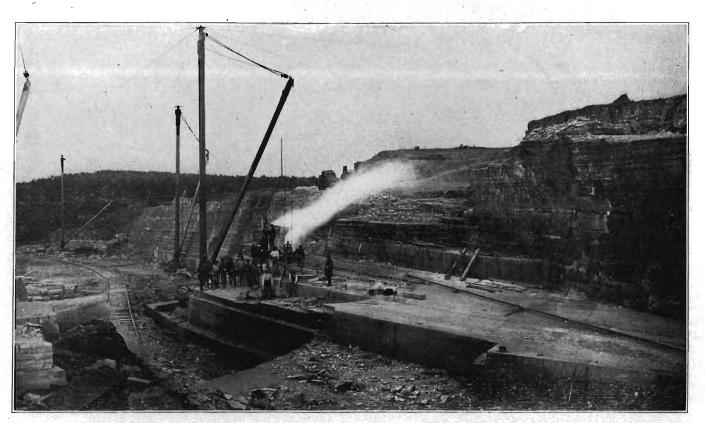
PLATE XXV-Champion quarry showing track and derrick arrangements and channeler. Stone City, Jones county. Crushed stone is the chief product at present.
