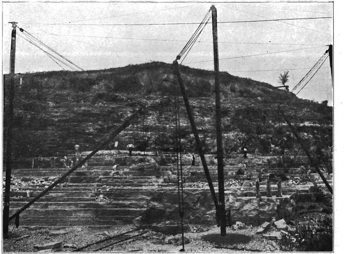
PLATE XXVII-State quarry, Anamosa, Jones county. This quarry is unique among the larger quarries of the state in the absence of improved machinery. All power is hand power.
