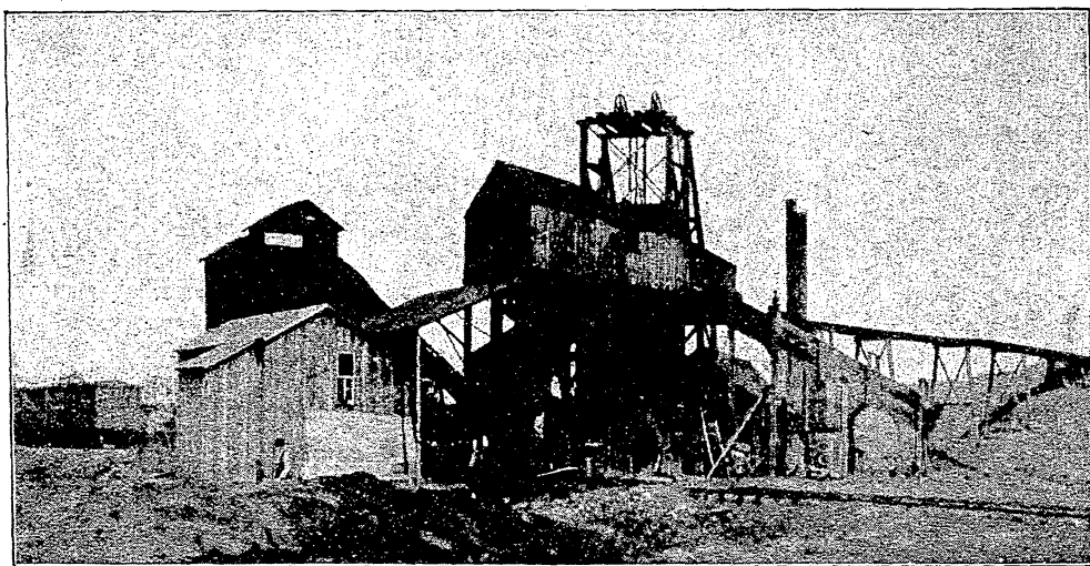
FIG. 24. Top works of the W. D. Johnson mine.
