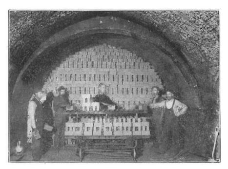
FIG. 72 Interior view of Haigh continuo is kiln showing method of setting brick; Sioux City Brick and Tile Company, Sioux City Iowa.
