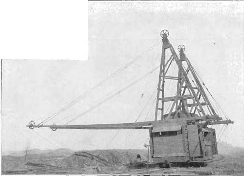
FIG. 76. Burnt clay ballast machine used by the Davy Burnt Clay Ballast Company.
