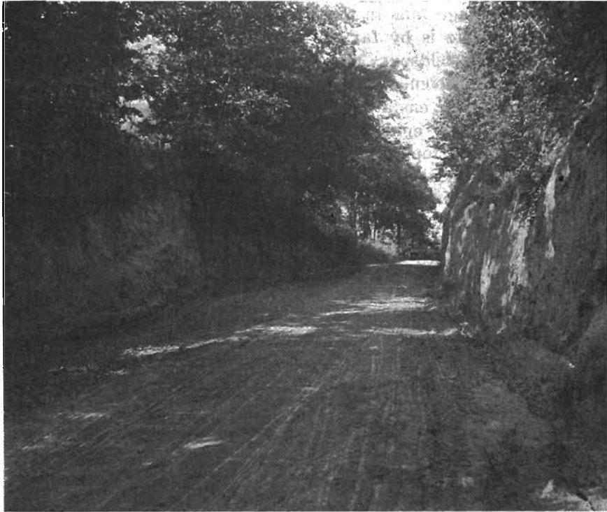
Figure 54. Vertical walls in a Peorian loess cut near Magnolia, Harrison County.
