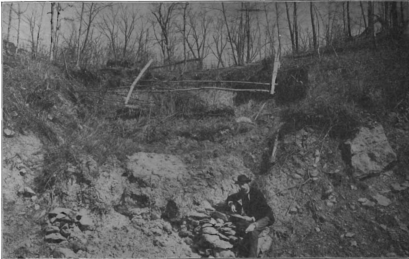
Mud flow of Independence shale, Linn section, Linn county. A wall built to confine it is now overflowed.
