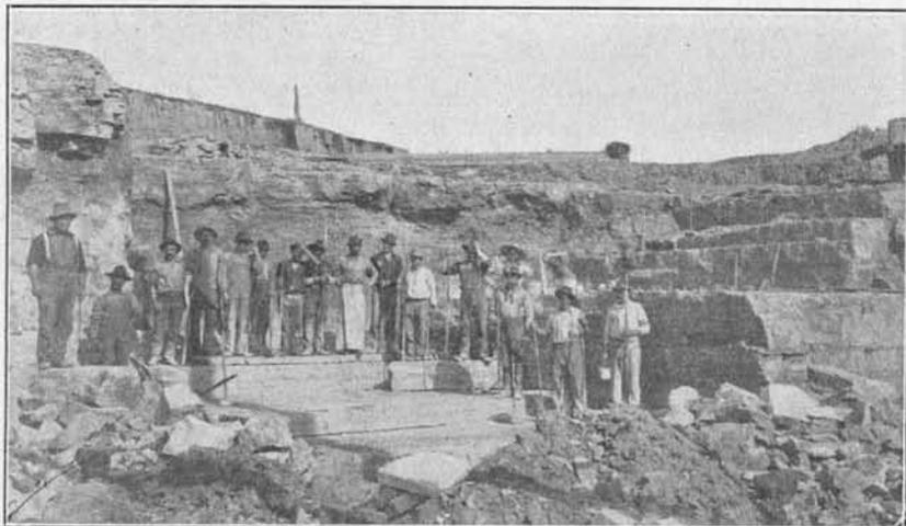
Fig. 52. East Farley quarry showing the characteristics of the Lower Quarry beds of the Niagara limestone.
