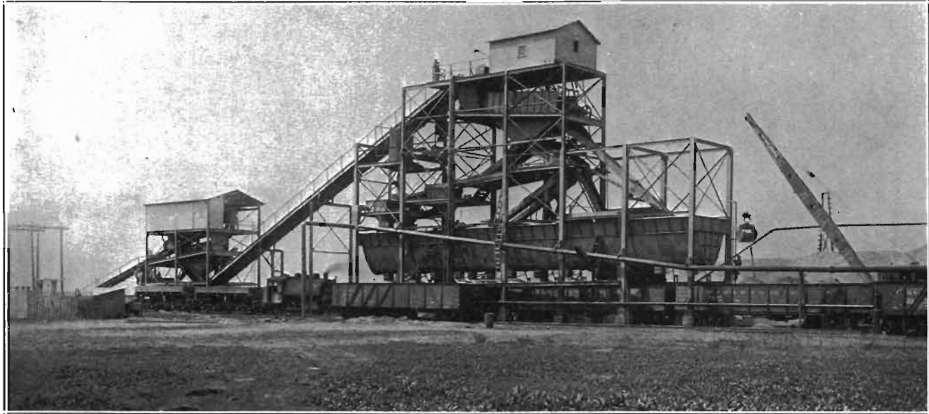
FIG. 32. — Gravel screening and washing plant at Hawarden. Courtesy L. G. Everist, Inc.
