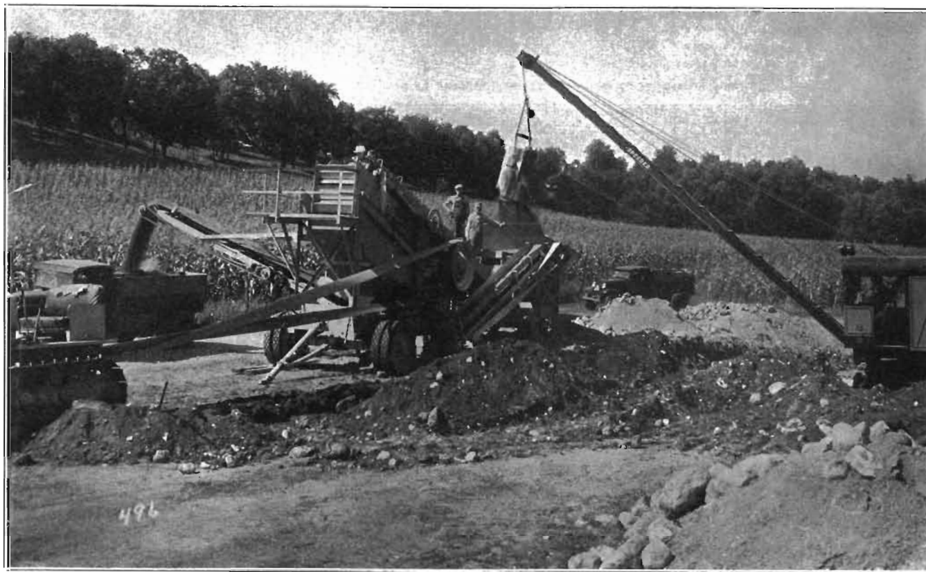
FIG. 33. — Portable surfacing gravel plant. Courtesy Iowa Manufacturing Co., Cedar Rapids.
