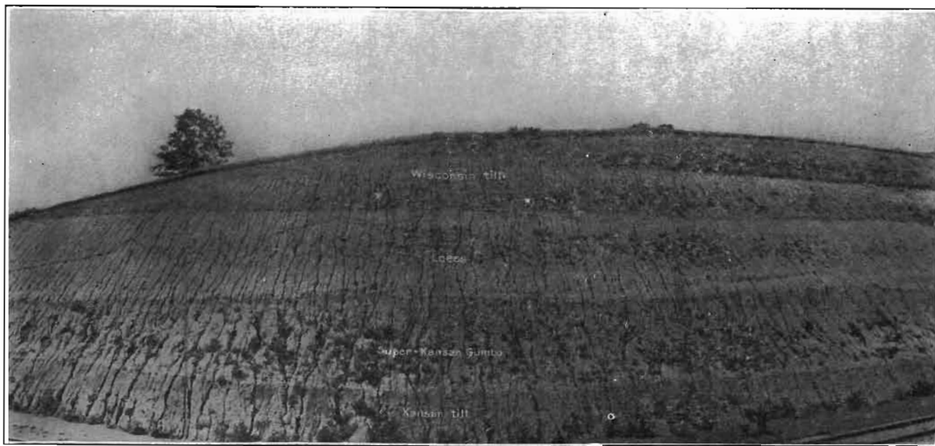
FIG. 54.—Cut southwest of Rhodes, Marshall county, showing Wisconsin till, loess, Kansan gumbo and Kansan till. (W. C. Alden.)
