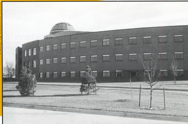
The Renaissance Design Group, a Des Moines architectural firm, designed the "geode building" in the late 1980s.
