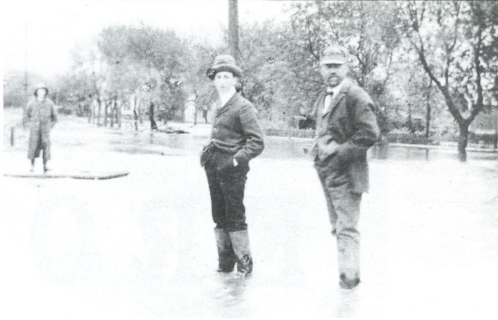
Leonard Hentges (left) and his uncle Nicholas Hentges of LeMars inspect the street corner where their house once stood. Heavy flooding in 1900 washed it away.
