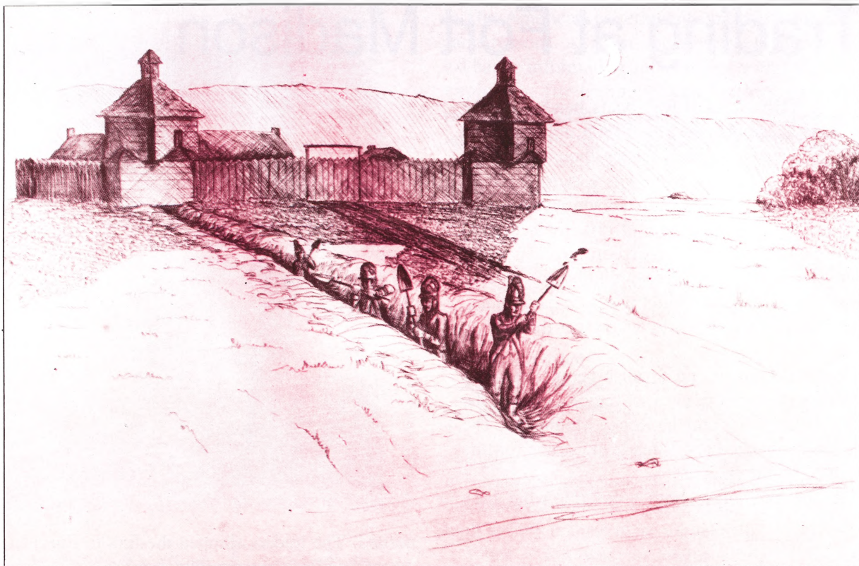
Soldiers dig a trench at night to escape from Fort Madison.
