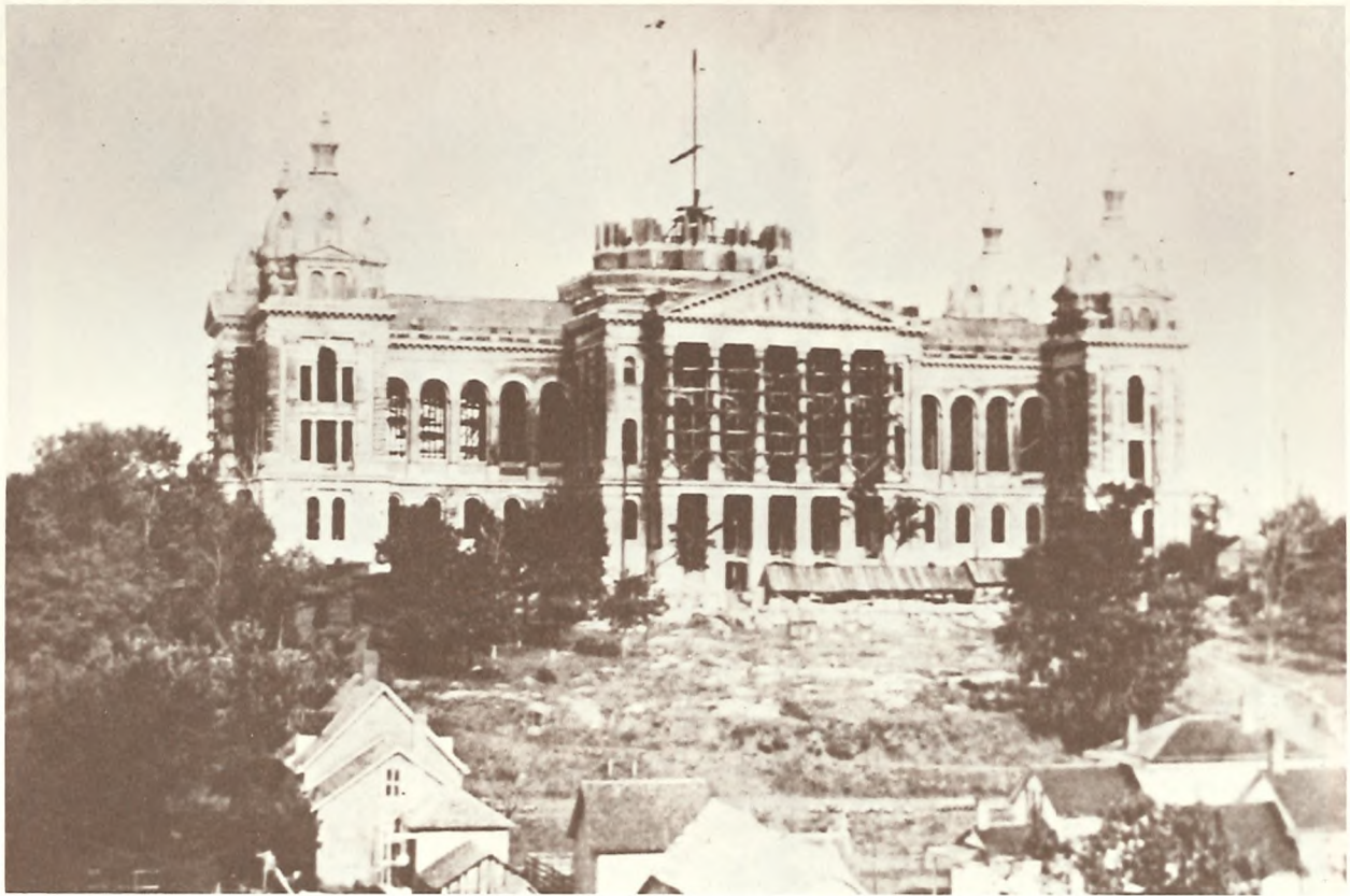
The dome begins to rise during the construction of the capitol, 1880.
