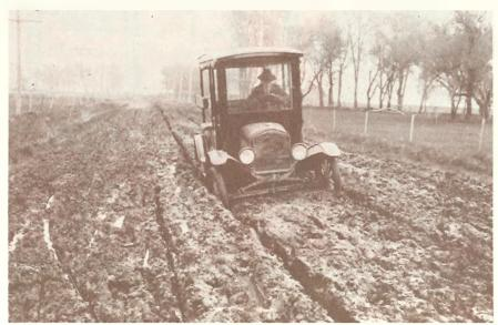
A motor truck on the Lincoln Highway (now U.S. 30) between Ames and Nevada, in 1918. Because the road was improperly drained, the road's gravel surface did little to improve it over a plain dirt one.
