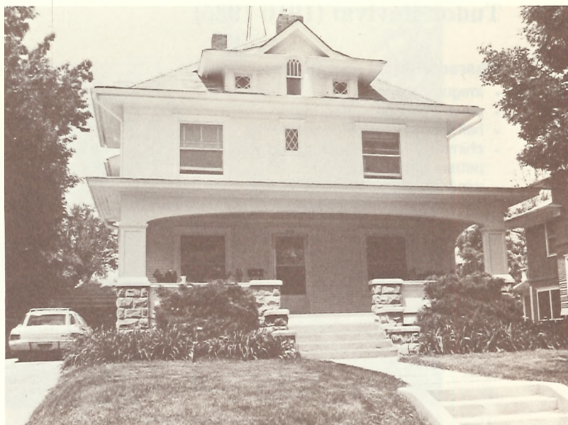
This basic house has a pointed Gothic window inside a pointed dormer. This is a detail borrowed from the past.
