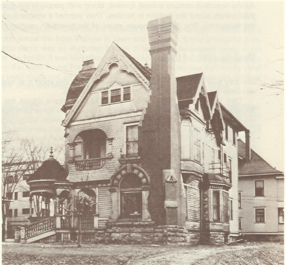
This Queen Anne style house was built from mail-order plans that cost $5. It is decorated with a little bit of everything. The walls are covered with stone, brick, fish-scale-shaped shingles, and wood siding. How many different types of windows can you find?
