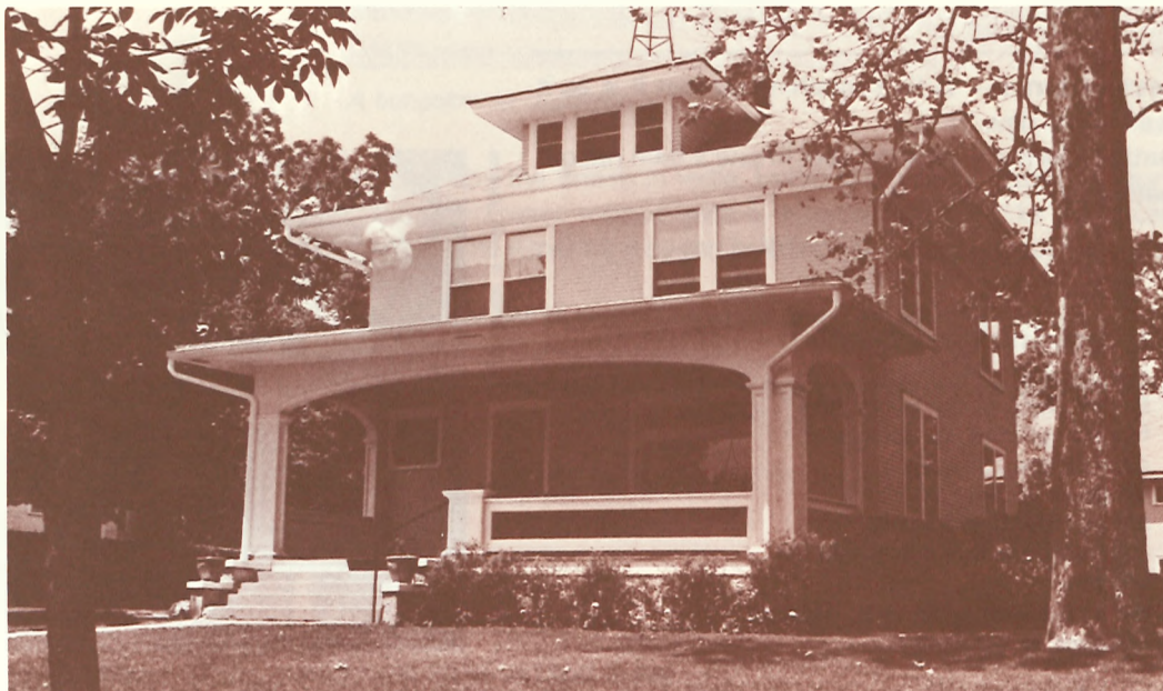
The dormer on this house has a flat top and a row of windows inside the dormer. This detail shows a Prairie style influence.
