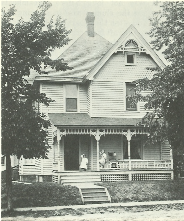
This house in Red Oak shows how milled wood products were used on homes.
