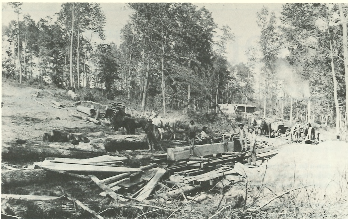
This early steam-powered sawmill was busy even before a roof could be put up.
