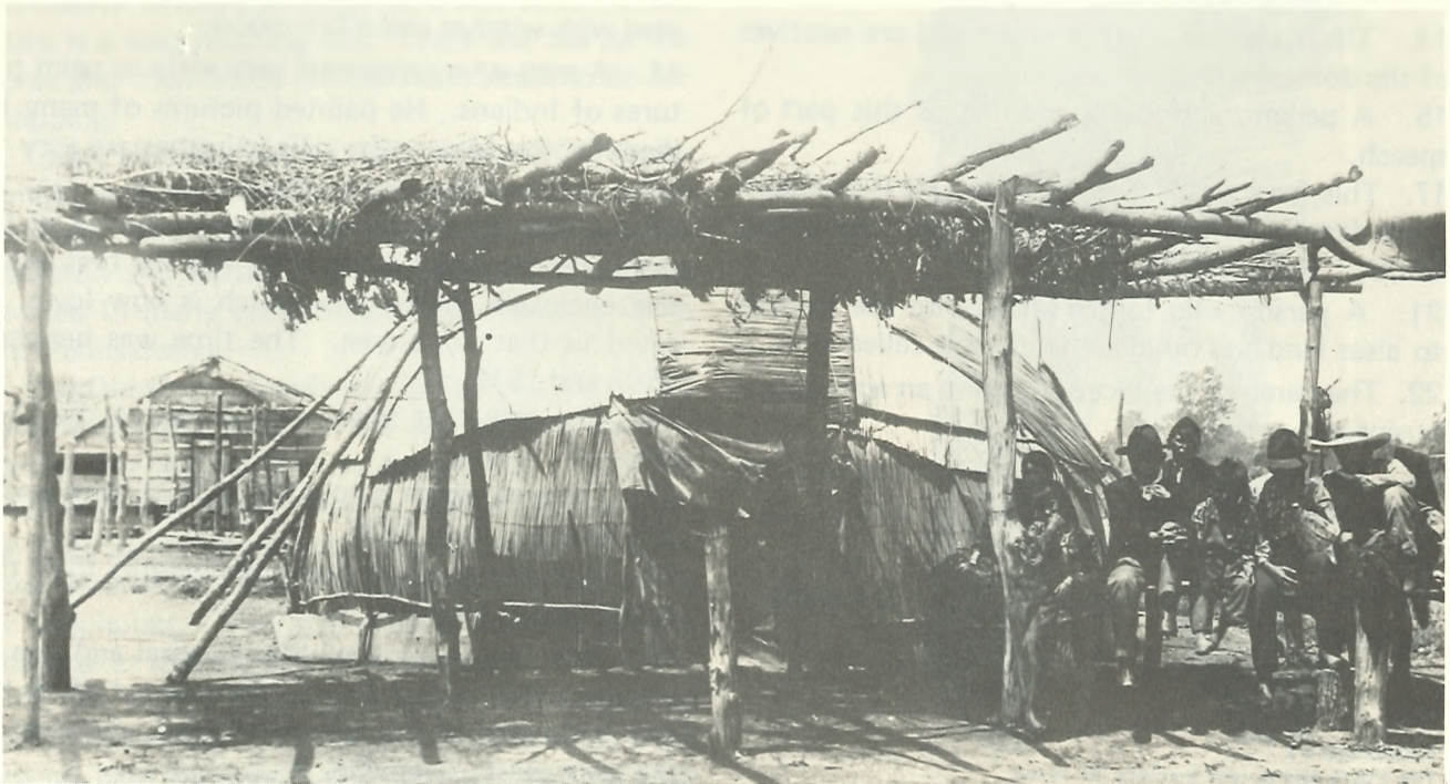
A Mesquakie house, called a wiki-up with a summer shade roof in front.
