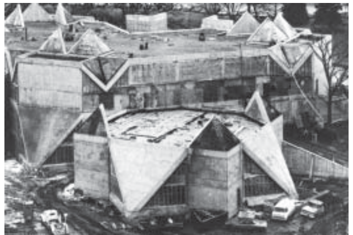
Health Sciences Library under construction, 1973
