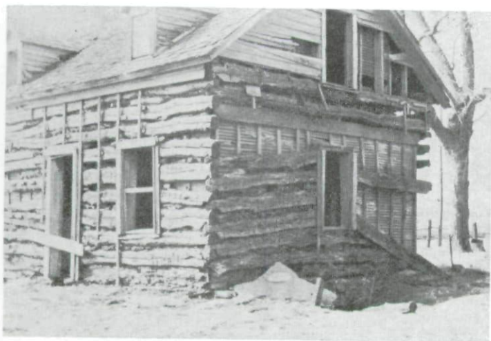
Southeast Corner of Cabin
