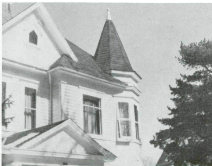
Gable Over Porch on South Side
