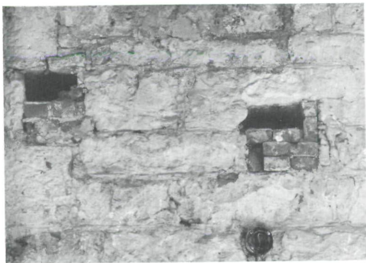
Figure 2. Brick-filled sockets in the interior stone wall indicate the positions of supporting beams for the gallery in the House Chamber.
