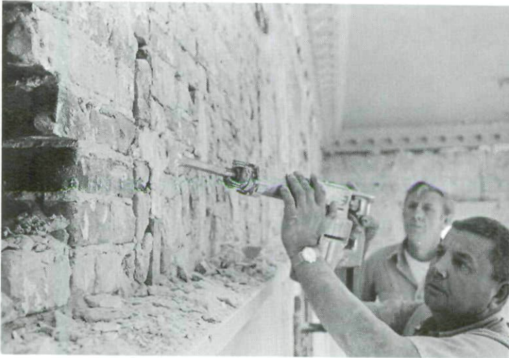
Figure 1. Dale Helfrich (foreground) and Tom Schoomer of The University of Iowa Physical Plant removing plaster from the interior brick wall of the House Chamber August, 1972. Photograph by Warren M. Paris.
