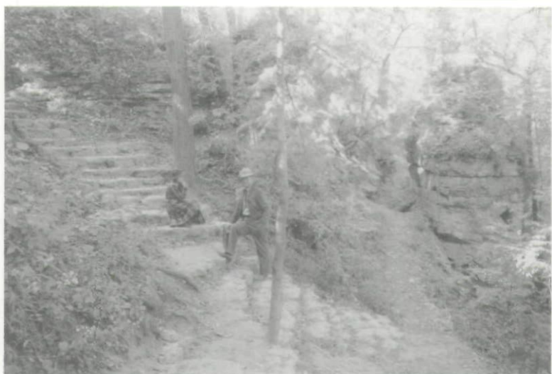
CCC crews began constructing the trail system at Backbone State Park in December 1933 and continued work for at least a year. Rough stone slabs were used to riprap hillsides in order to blend trails into the limestone outcroppings that characterize the park's natural landscape. Photo (c. 1940) courtesy of the National Archives.
