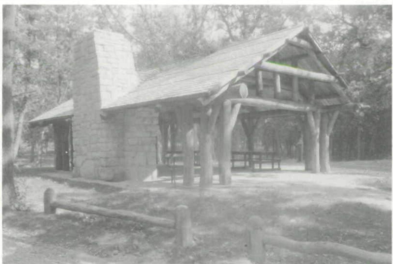
Picnic Shelter, Backbone State Park, constructed by the CCC between February and April 1935. Its location near the west entrance to the park was once the center of the park's camping area but now functions as a picnic spot. Photo (c. 1940) courtesy of the National Archives.
