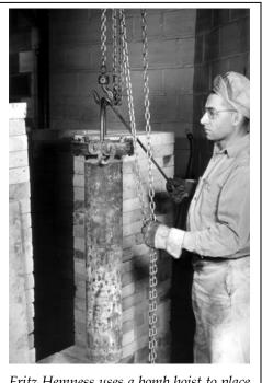
Fritz Hemness uses a bomb hoist to place uranium reduction bomb 399 in a gasfired furnace in the "Little Ankeny" building on the ISC campus, ca. 1942–1945.
