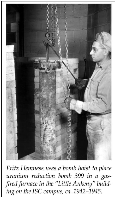
*Fritz Hemness uses a bomb hoist to place uranium reduction bomb 399 in a gas-fired furnace in the "Little Ankeny" building on the ISC campus, ca. 1942-1945.*
