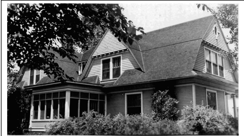
The author's family home at 605 Kellogg Avenue in Ames. In 1961 it was demolished to make way for an automobile repair shop. All photos courtesy of the author.
