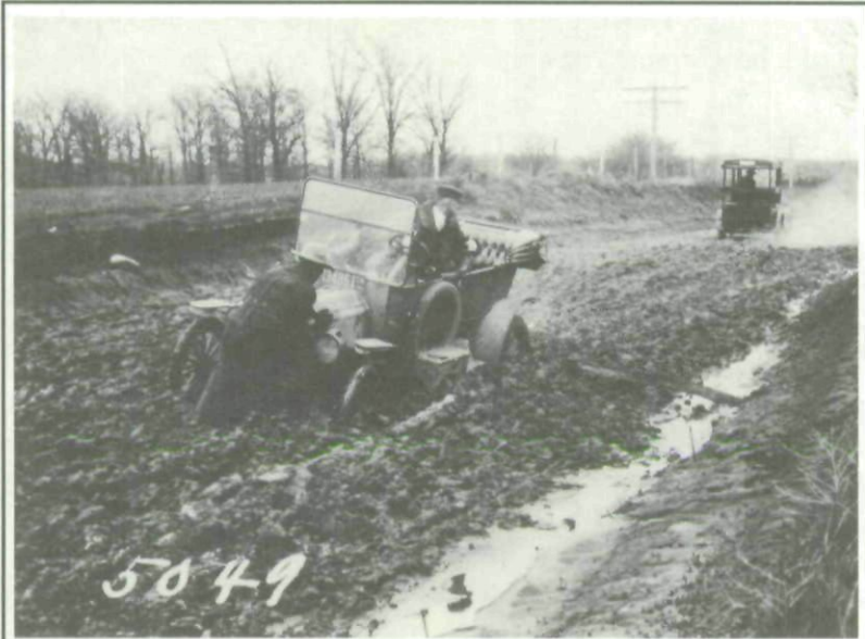
For motorists, Iowa was synonymous with "gumbo" in the pre-pavement days. Notice that this section of the Nevada Road, east of Ames in Story County, appears to be entirely below the natural grade. Photo c. 1917, courtesy Iowa Department of Transportation.
