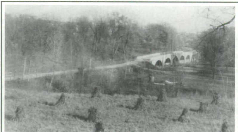
This view of the Eureka Bridge, located three miles west of Jefferson, c. 1920, would now be obscured by dense vegetation on the hillside. Constructed in 1912, the concrete deck-arch bridge was designed by bridge engineer James B. Marsh of Des Moines, who is noted for his distinctive "rainbow arch" bridges. Courtesy Iowa Department of Transportation.
