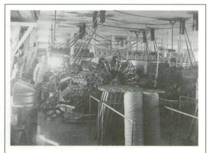
Two workers pose with equipment in the woolen mill's carding department. The rolls of material in the foreground are "roving" that has been through the carding machine and is ready to be taken to the spinning machinery. The carding machine is the large piece of equipment with all of the rollers in the center. Photo, 1899, courtesy of Arthur Selzer.
